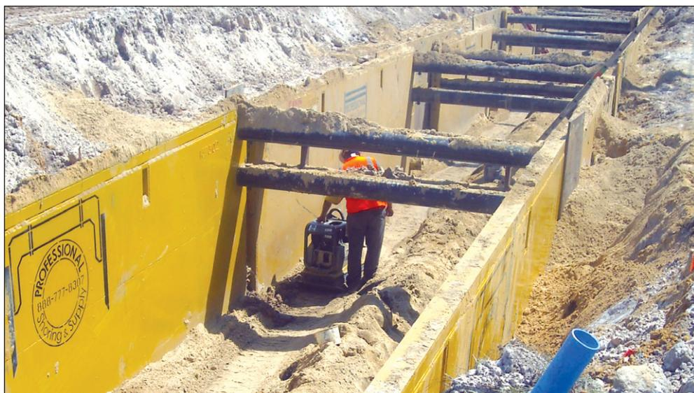
To facilitate the protection of workers fitting pipes in trench excavations, RIPA employed a series of Efficiency Production manufactured trench shields, also known as "trench boxes," to shore the pipelines.
