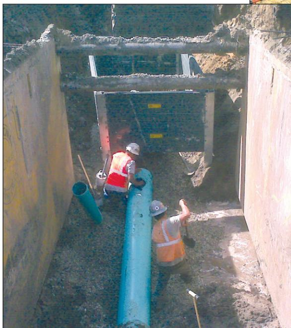
RIPA utilized a 4-sided modular aluminum Build-A-Box system from Efficiency Production to tightly shore around the installation of precast manholes.
