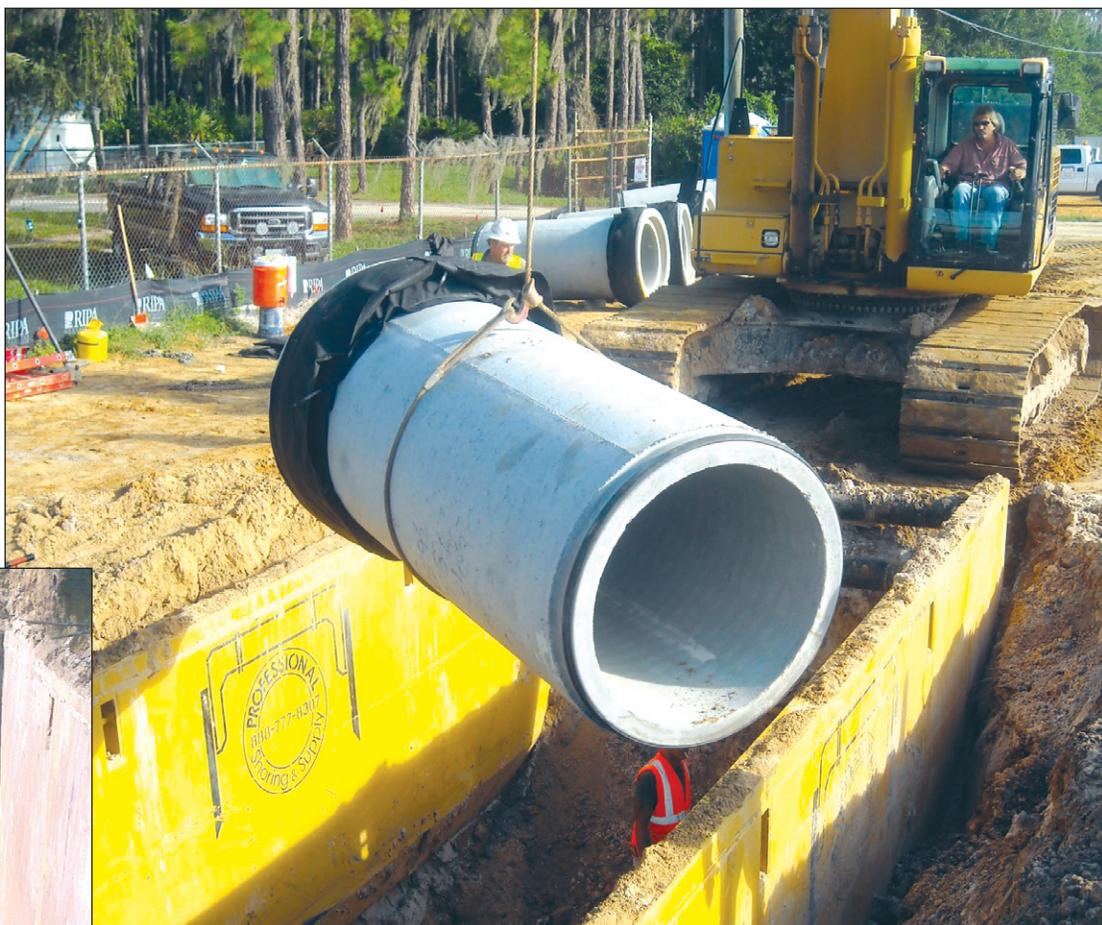
RIPA installed several types of RCP pipe for water, and sanitary and storm sewer. The largest diameter pipe is 72 in. (183 cm) in 10 ft. (3 m) lengths.
